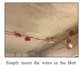
Splice slots, compress the button on
