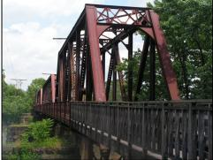
ight next to it, was a marker dedicating the Harmar Bridge, one of the last Pratt through truss bridges, with a swing bridge on the far section: The Harmar Bridge was originally an old covered bridge and converted to a railroad bridge back in 1873 for the B&O railroad
